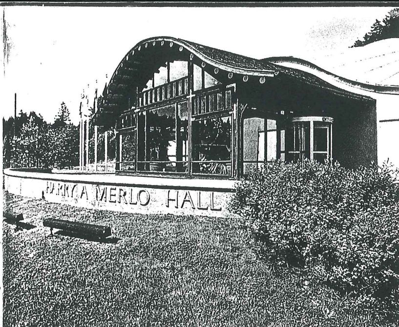
Vista externa do WFI / External view of WFI
